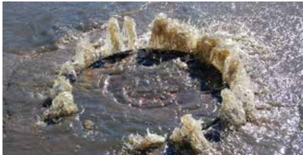
When sewer lines get plugged and cannot direct raw sewage into the treatment plant, it can cause overflow onto the streets as shown in this overflowing manhole cover.
